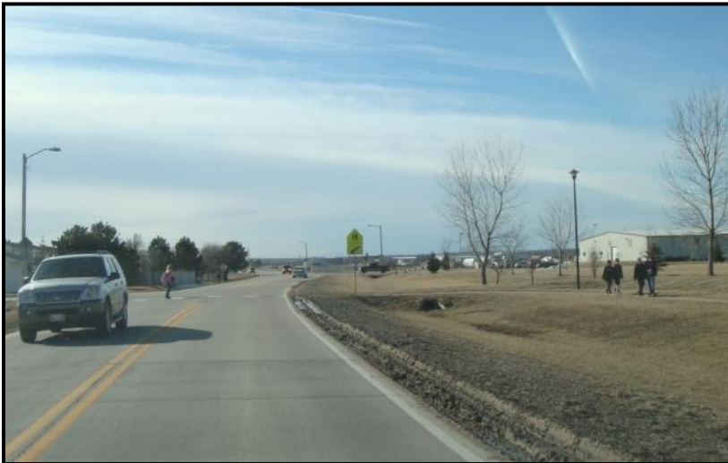
Amberly Road at 140 th Street - Westbound
