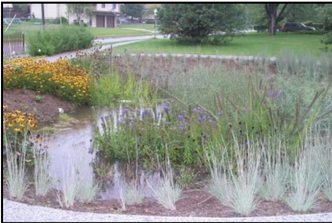
Typical Rain Garden / Vegetated Swale
