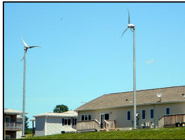
Net Metering Small Wind Energy Systems Winnebago, Nebraska
